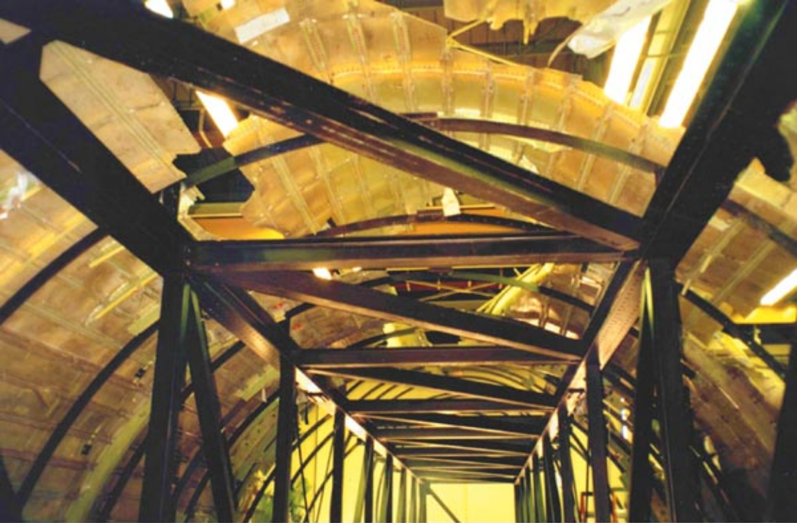
The roof of the plane from inside
