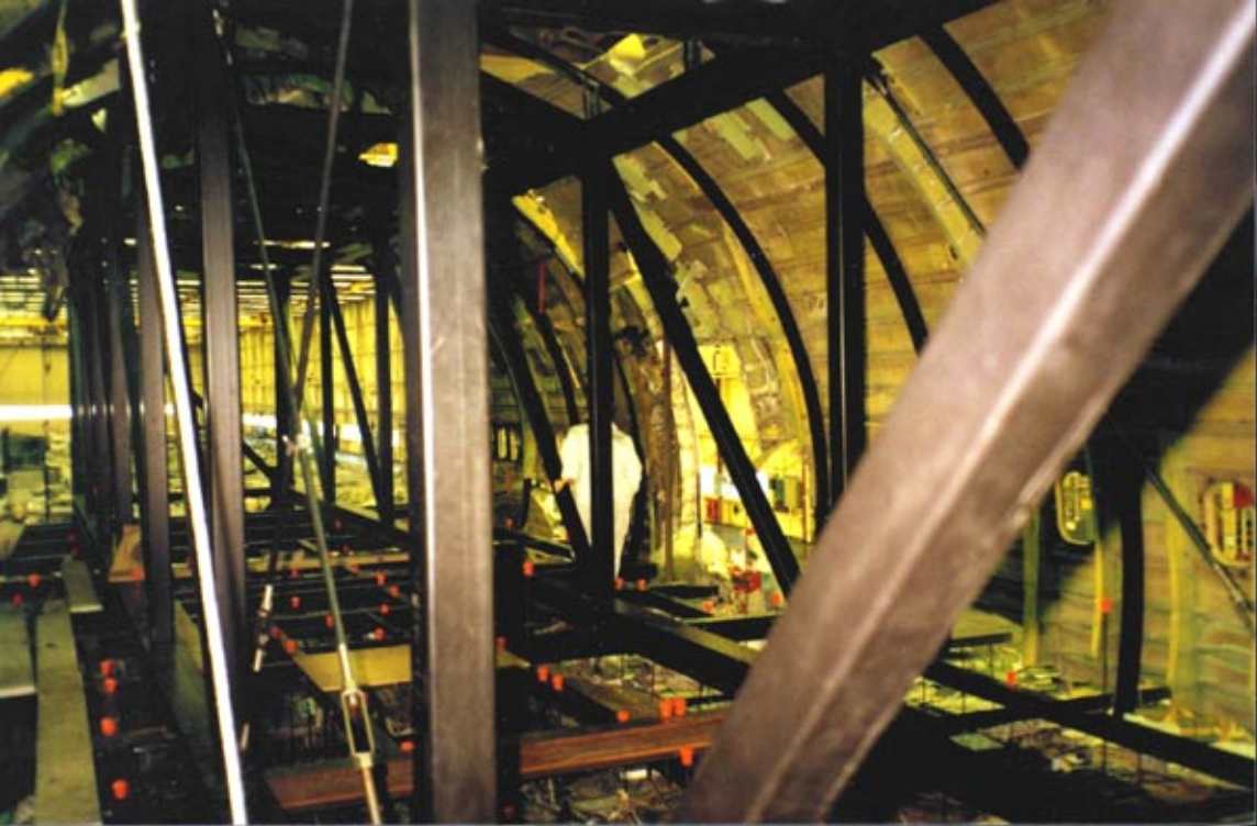
Internal view of the right side looking rearward
