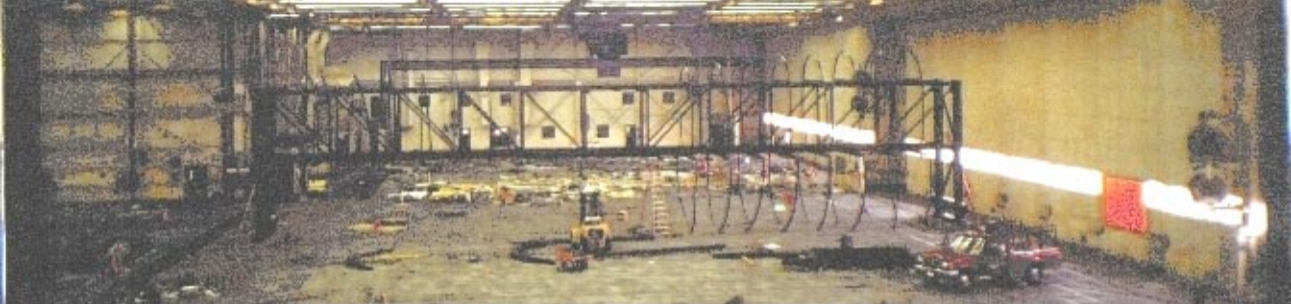
The truss assembled to support the piece of the plane on February 6
