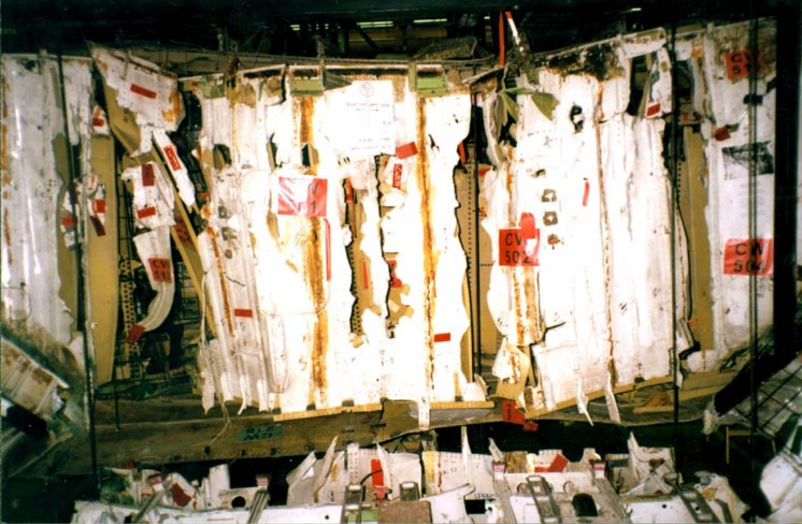
The front spar looking rearward
