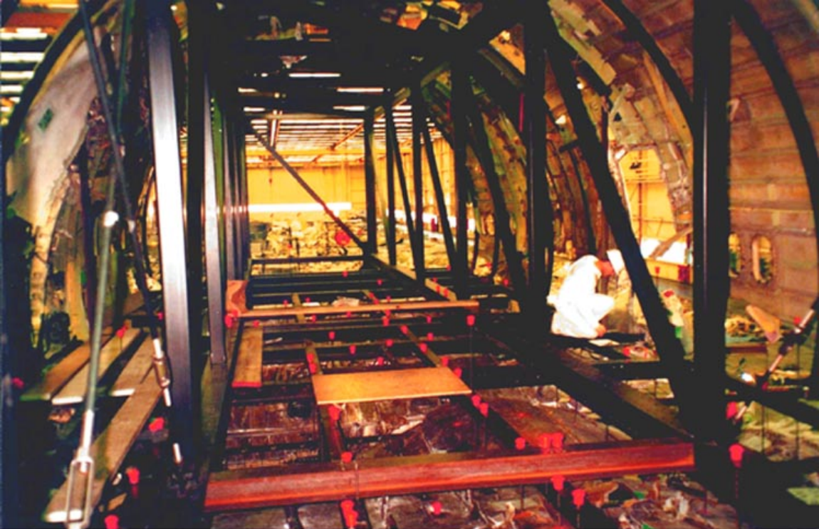
Internal view looking rearward
