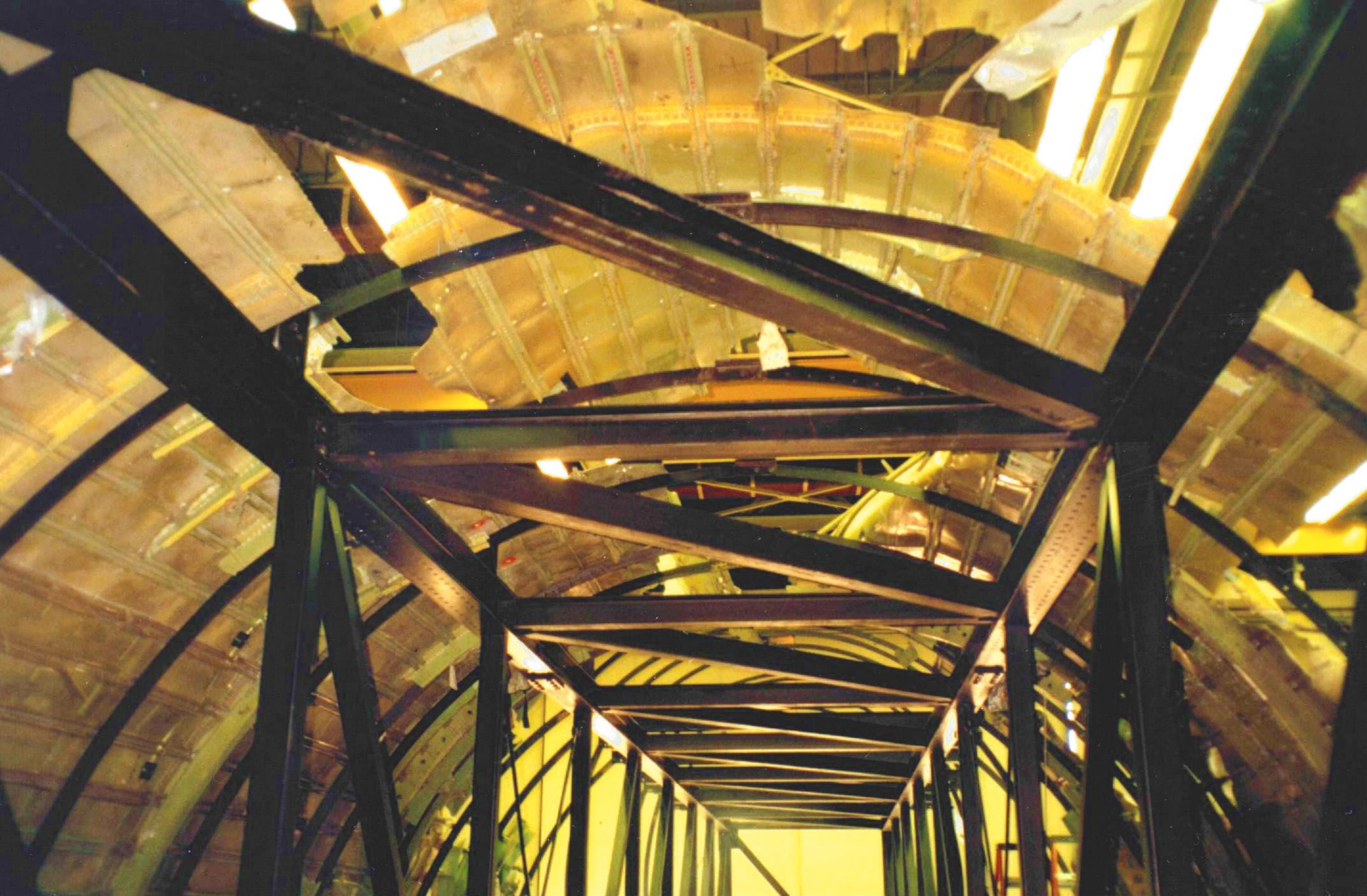
The roof of the plane from the inside
