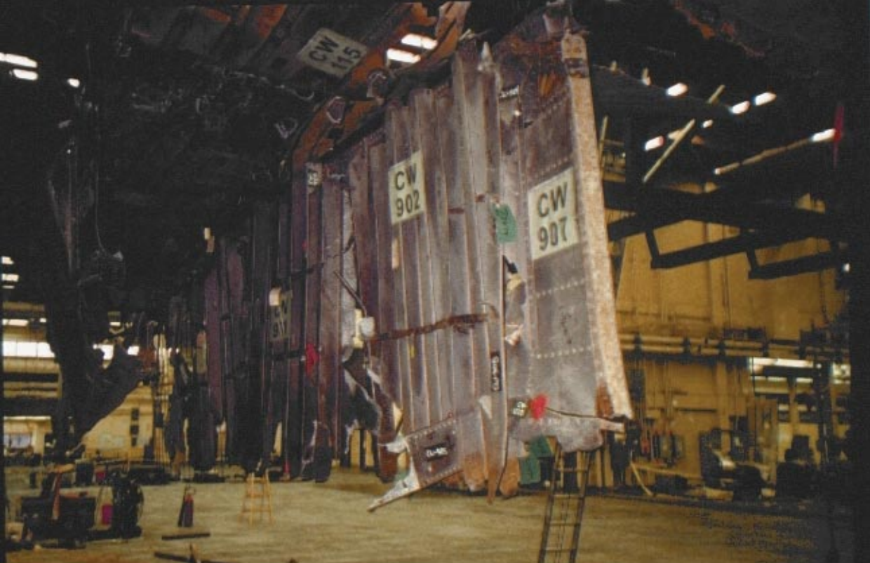
The left hand side of the front of Spanwise beam 1 as viewed from the side, looking at CW 902 and 907
