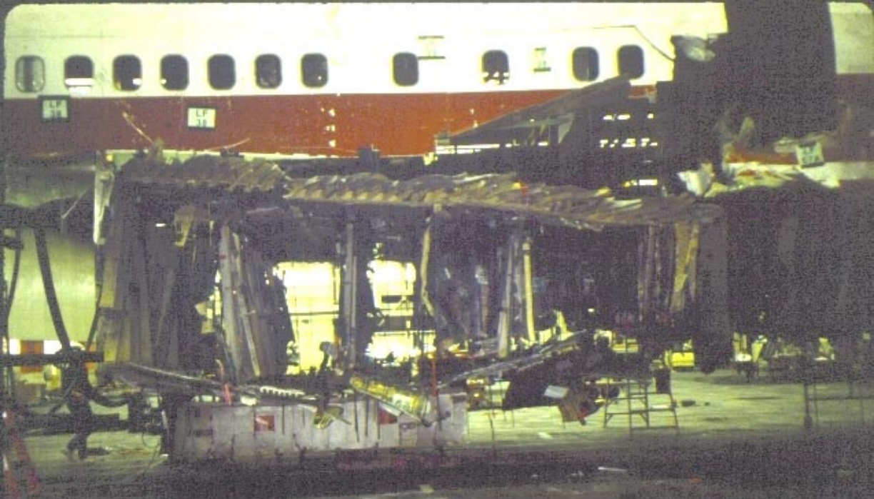
Left side of the center wing fuel tank with bottom floor and portions of the keel beam
