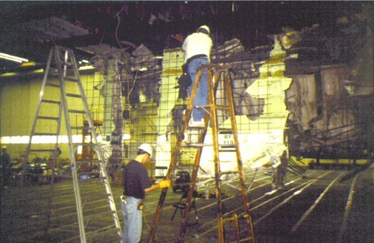
Working on the 1450 bulkhead on February 26 after installation of RF119
