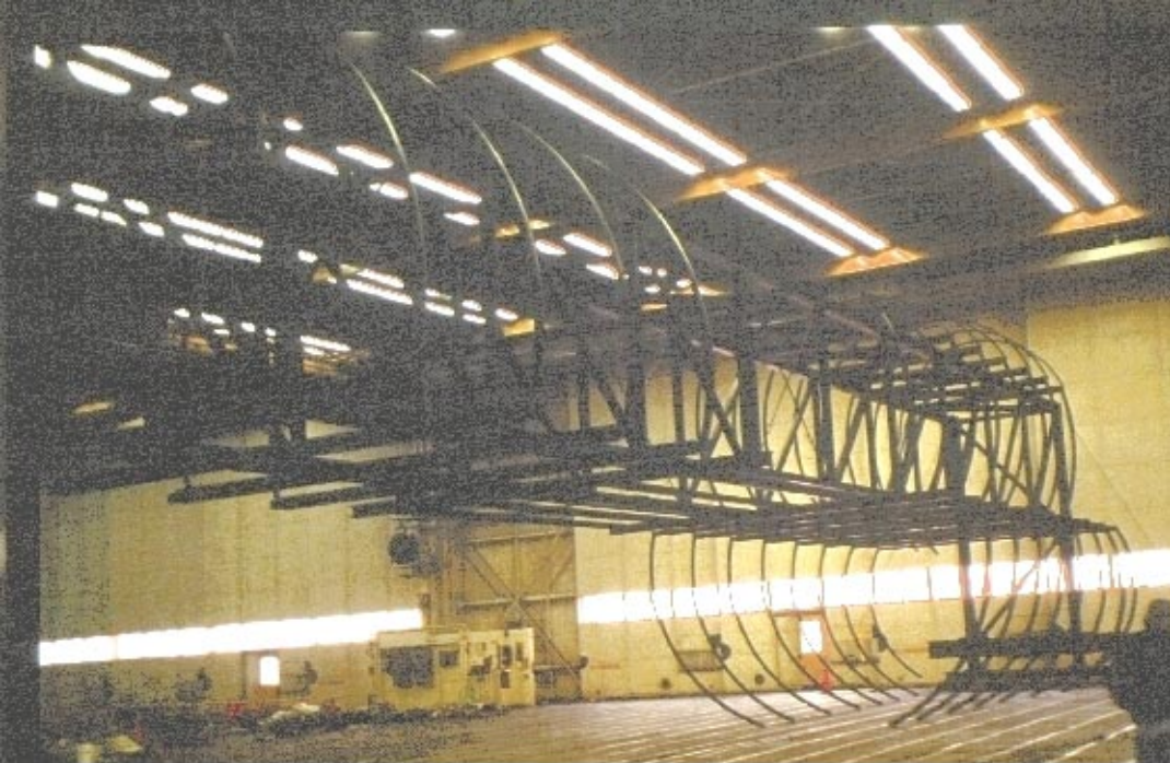
Close-up of the truss assembled, looking towards the front
