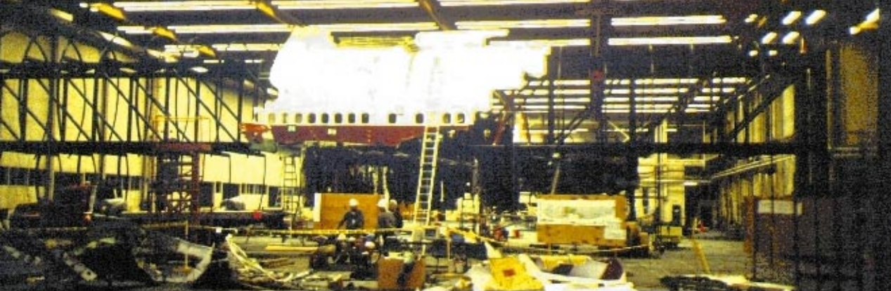
Installation of the remaining portion of LF 38 on February 20
