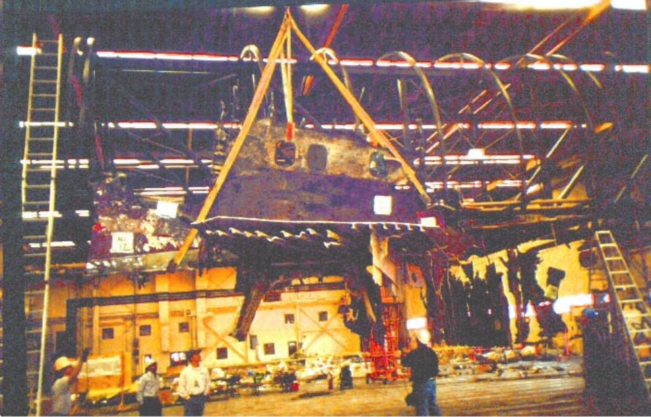
The truss assembled to support the piece of the plane on February 6
