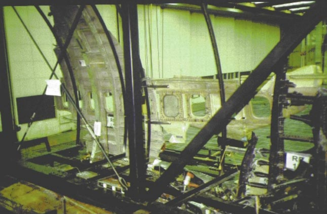
Looking at the right interior, including RF37, RF14, RF114A, and RF17
