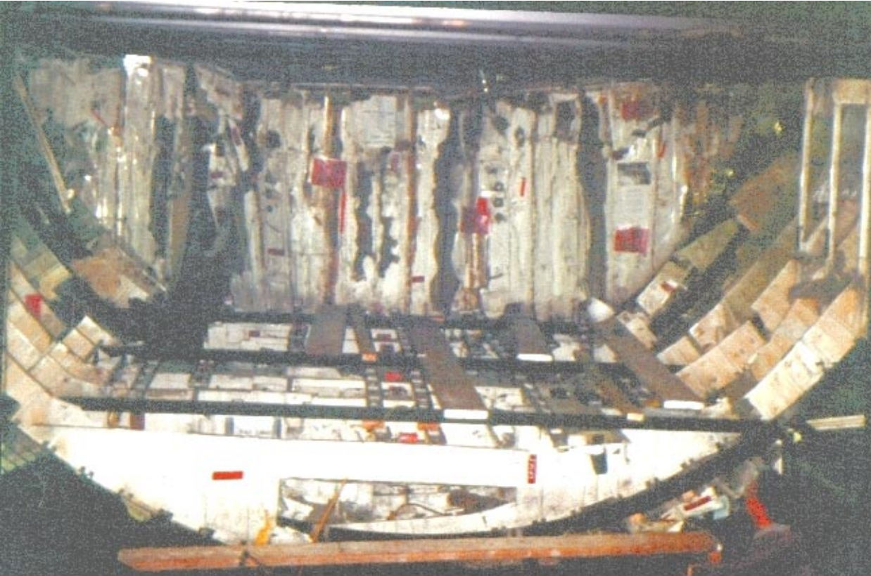
The front cargo bay prior to lowering
