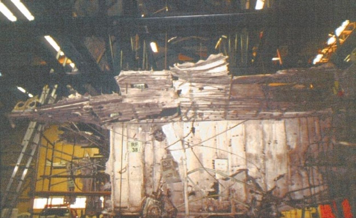
Looking at RF38, the 1350 bulkhead
