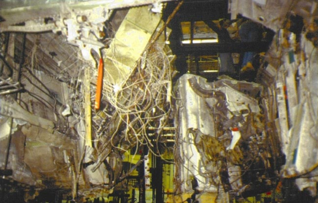
Looking at the pressure deck and LF40 from the right to left
