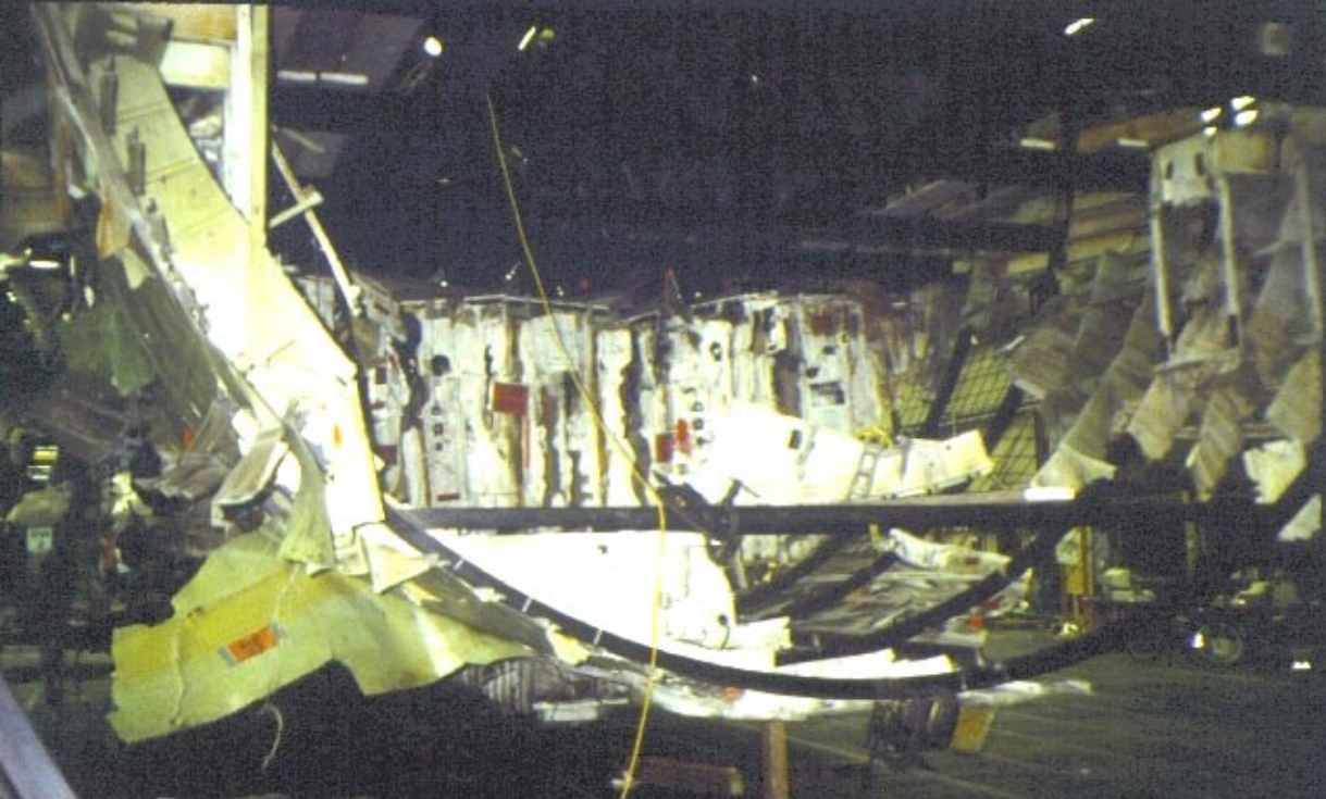
Building the front cargo bay area
