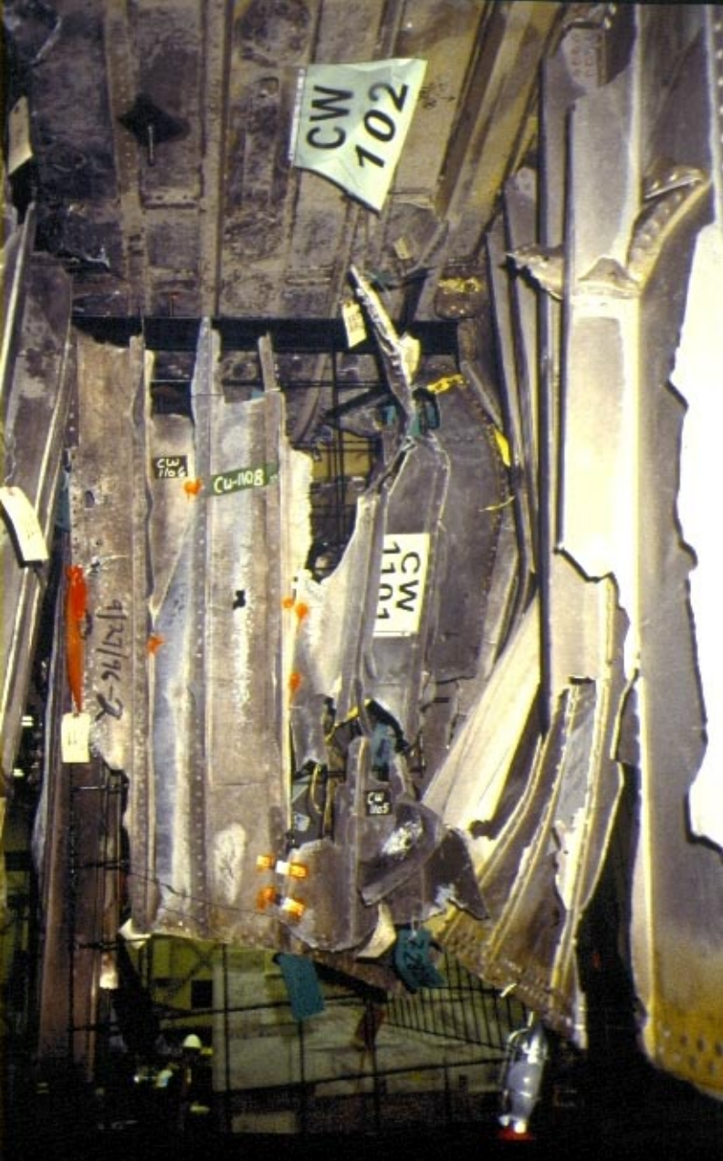
Looking at CW1106, 1108, and 1101
