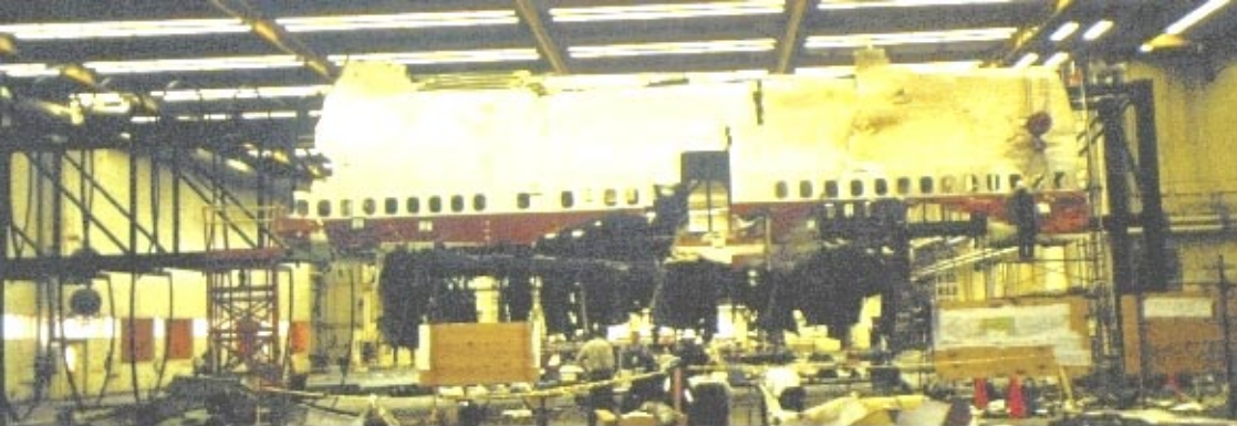
LF2 attached to the truss on February 26
