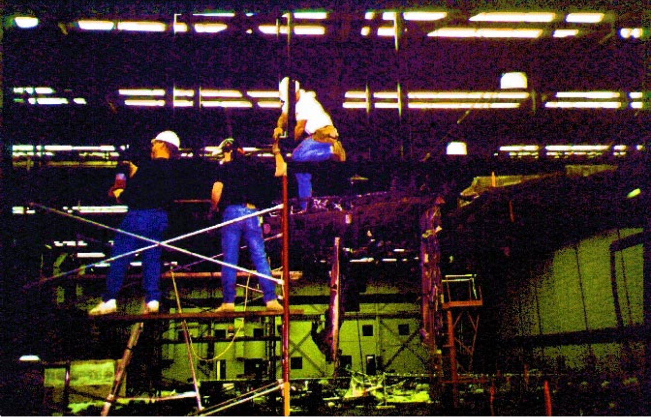
Crew working off scaffolding to assemble pieces
